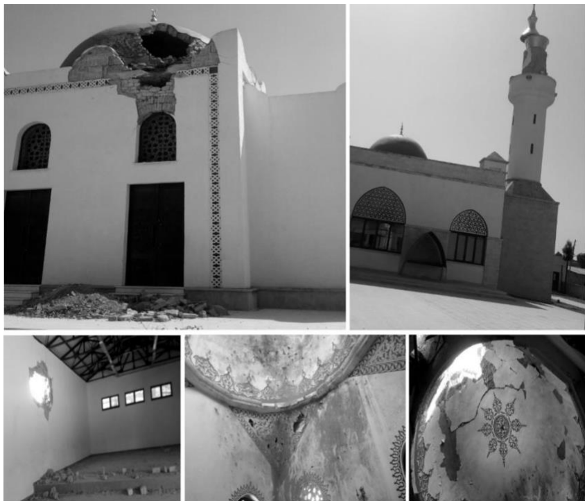
Figure 6.23. The exterior and interior surfaces of Al Nejash Mosque, minaret and the mosque's hall which are severely damaged by shelling
