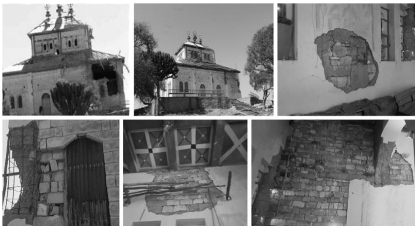
Figure 6.8. Destructions of Qirqos Church building (upper left) (Source: social media), interim conservation works carried out by the local communities in the interior and exterior surfaces of the church building
